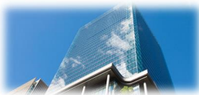
Grand Front Osaka Tower B 27th Floor
