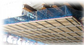
System hanging scaffolding VMAX
